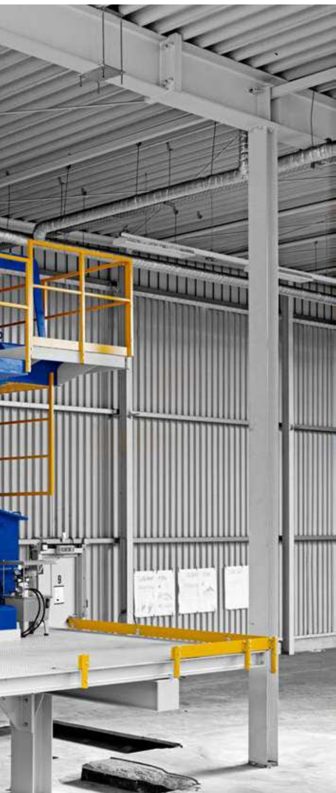
Rotorshredder of type 2018 during construction of an E-Scrap recycling plant.
