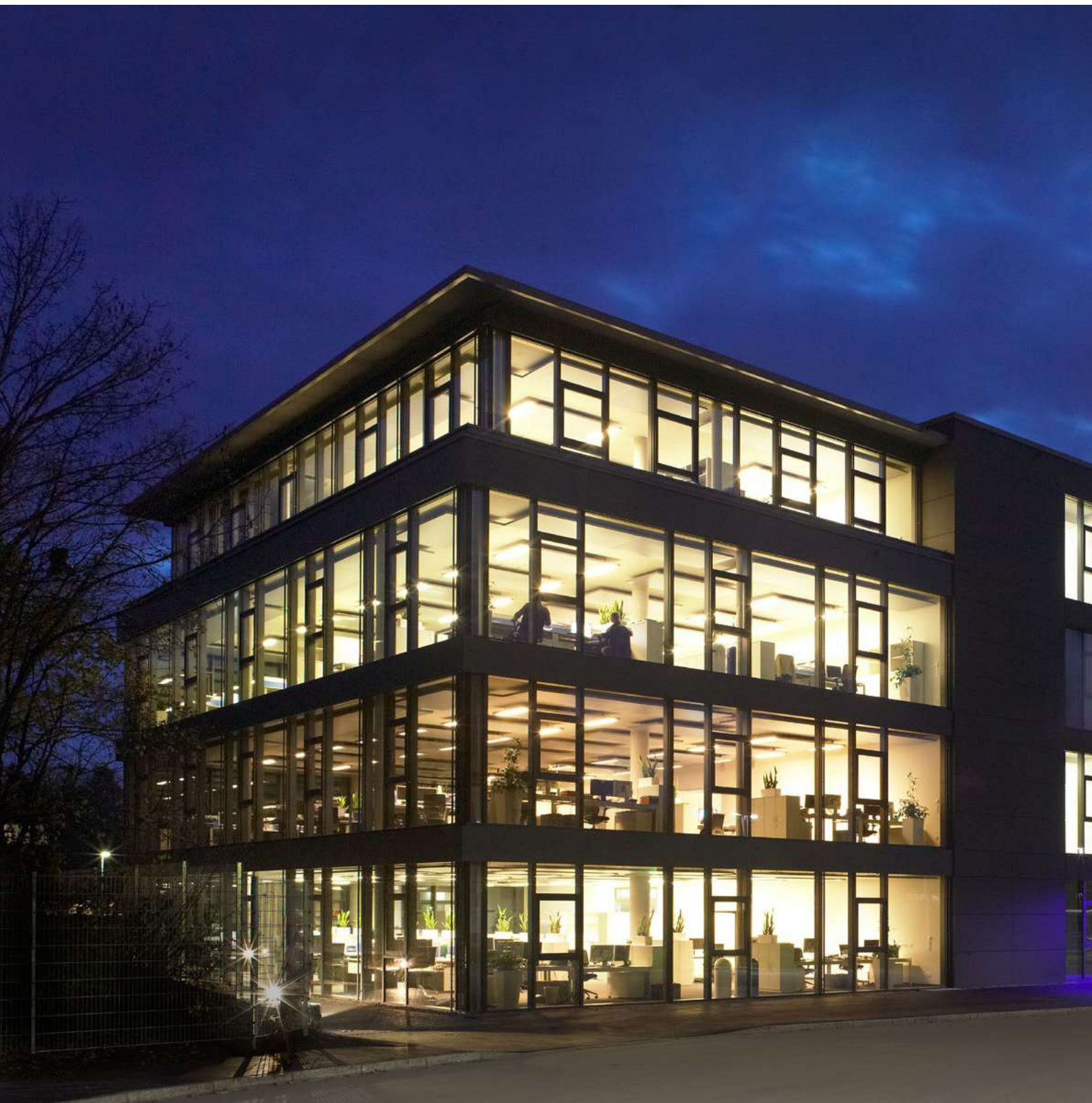
Office building at BHS-Sonthofen
